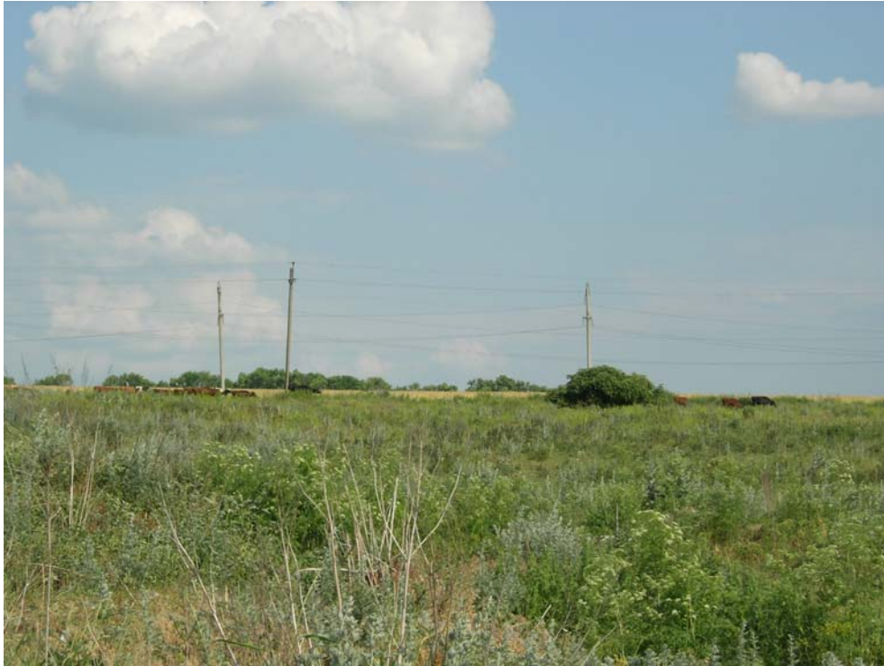
Picture 3 Very high voltage line
