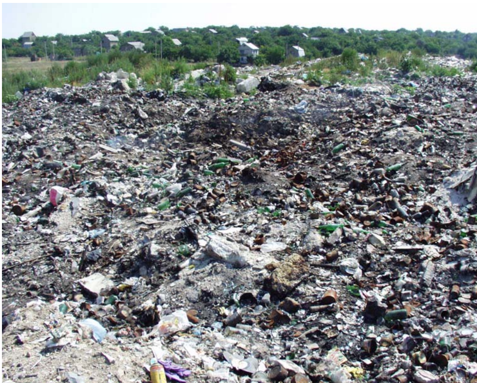
Picture 35 Simferopol Landfill: Self combustion of the waste
