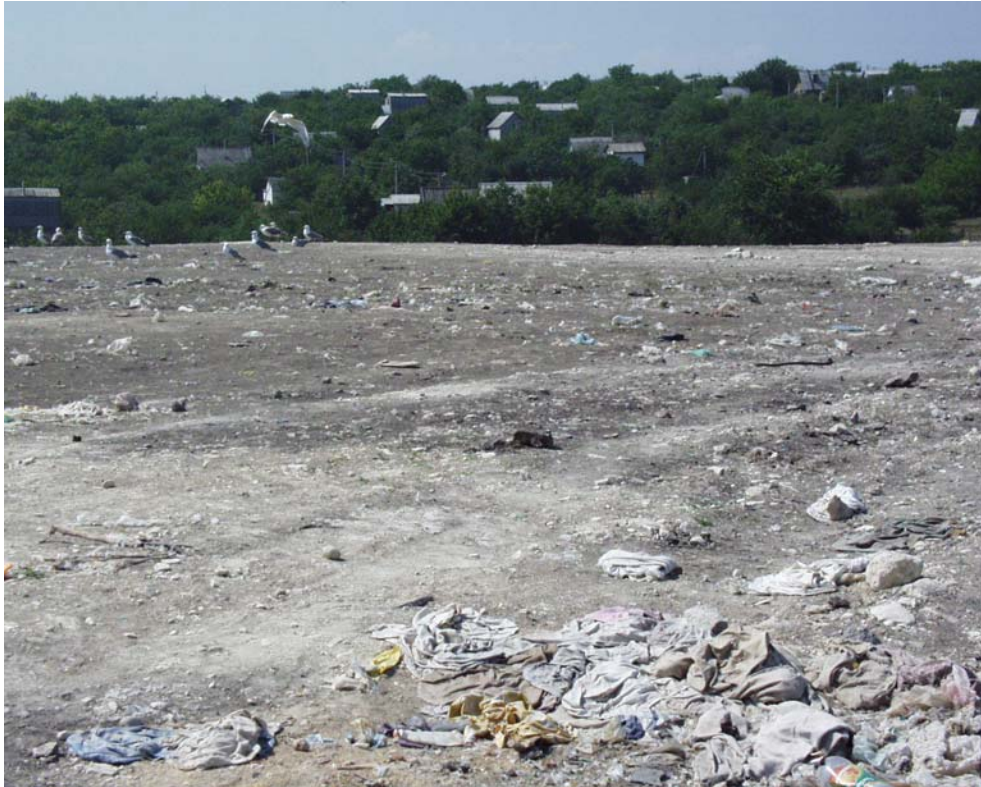
Picture 41 Simferopol Landfill: Cover with construction waste
