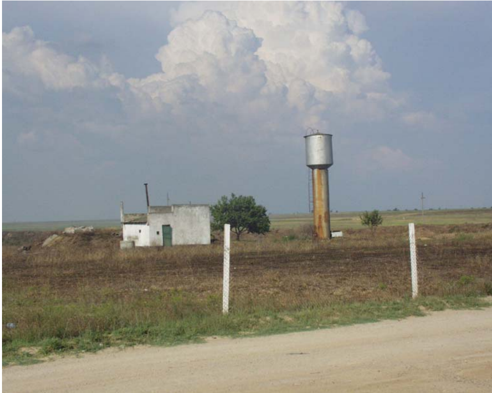
Picture 13 Evpatoria Landfill: Place of the water supply borehole
