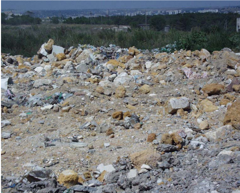
Picture 39 Simferopol Landfill: Cover with construction waste
