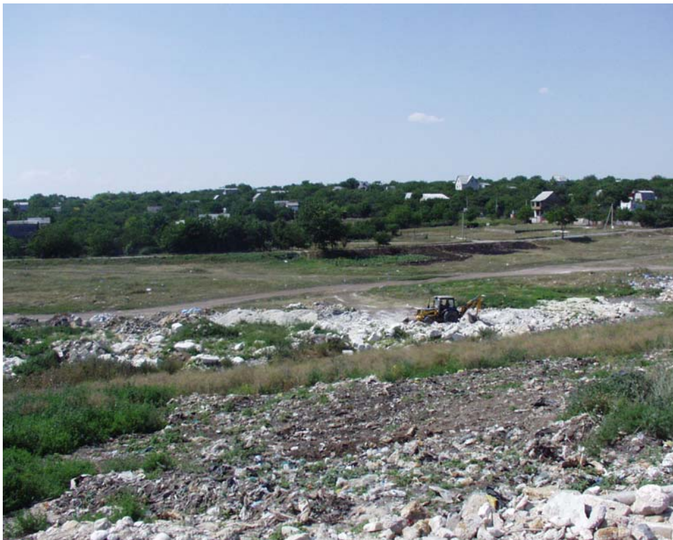
Picture 42 Simferopol Landfill: Cover with construction waste
